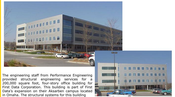
consists of auger cast pile foundations, slab-on-grade, composite steel-framed floor slabs, and steel-braced frames for lateral load resistance. The roof structure design included provisions for the building's mechanical equipment and enclosures. The structural analysis of this building included a complete floor vibration assessment of the composite floor system.
